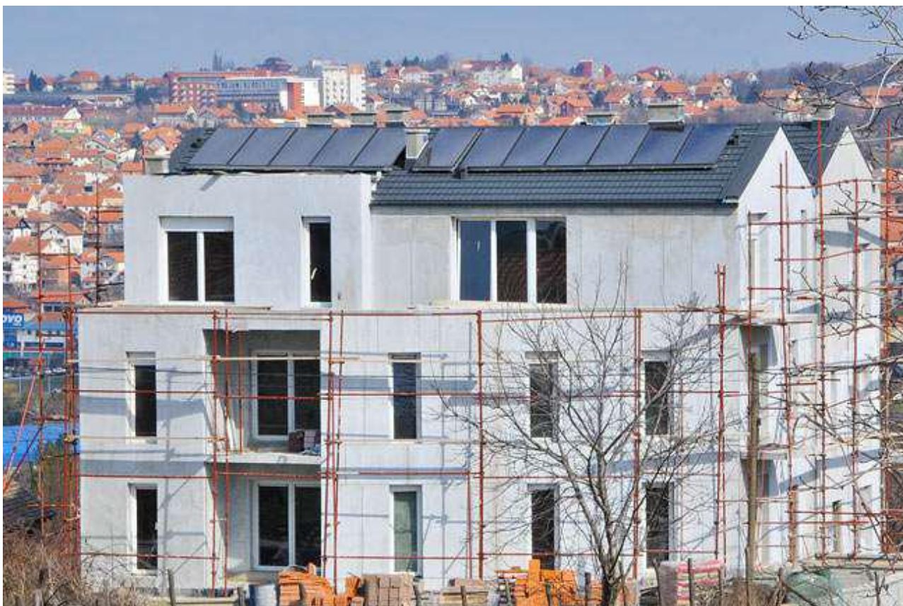
Baumit PutzSpachtel ant fasado (foto Beodom).
